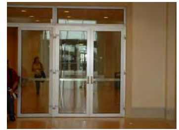
Aluflam one hour fire rated doors and framing system installed at FIU School of Law—Miami, FL
